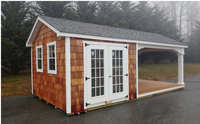
A-frame style enclosure with vinyl pavilion deck, cedar shake siding, composite deck flooring
