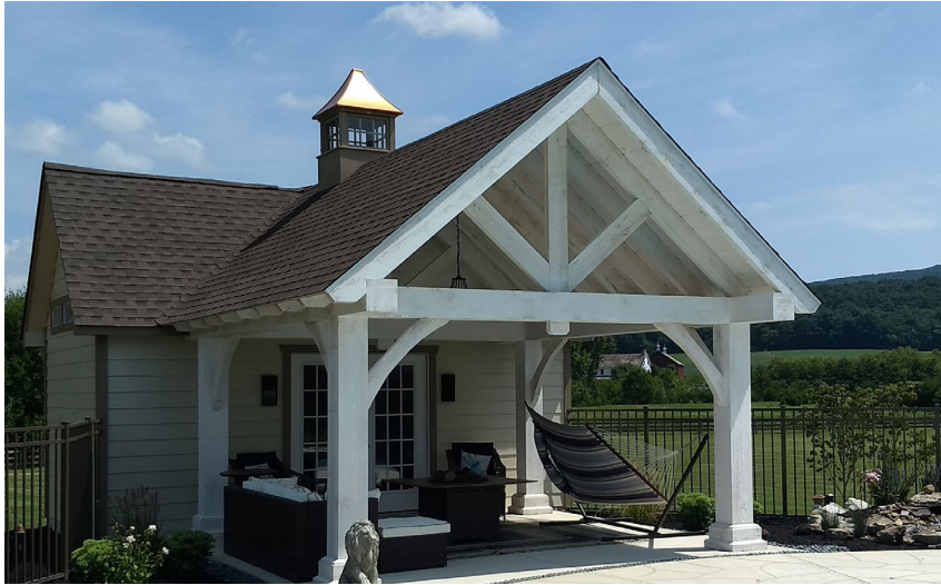
Open gable A-frame style, painted wood material, shingled roof, exposed rafters, studio enclosure addition
