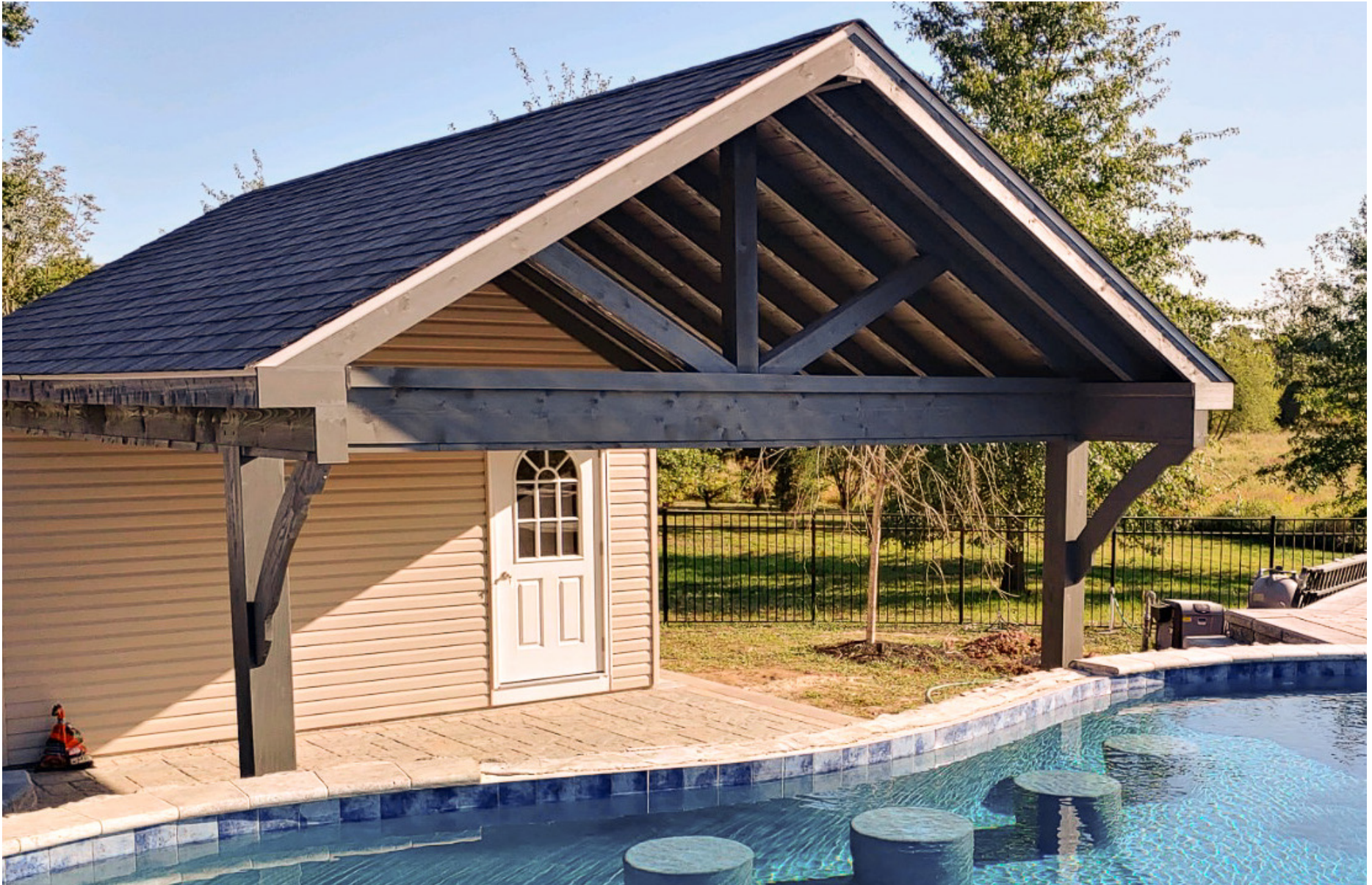
Open gable A-frame style, stained wood material, shingled roof, storage closet addition
