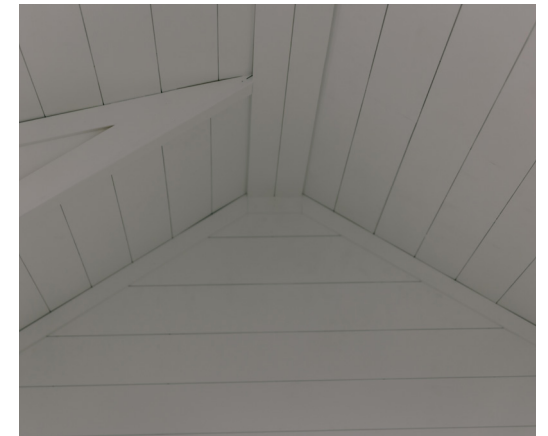
Nickel gap ceiling
